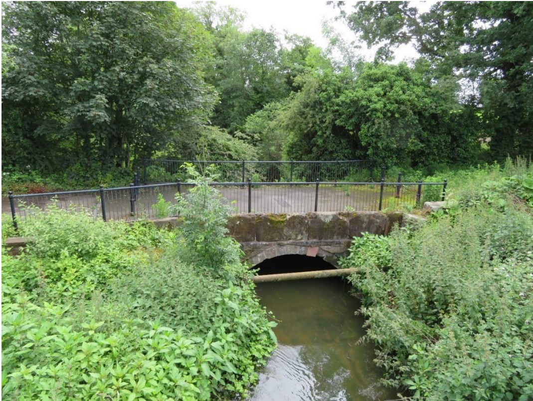
Plate 41 Warburton Lane Old Bridge
