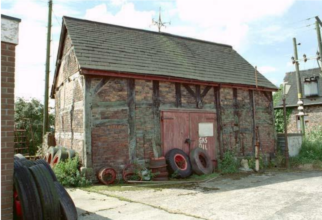
Plate 27 Timber framed building at Warburton Park Farm, taken in 2001 © IoE F.
