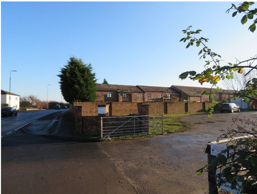
Plate 14 Looking south-east towards the barn at Ackers Farm. This blocks any views towards the farmhouse
