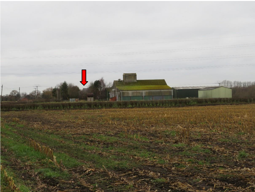
Plate 22 Looking north-west from Moss Lane towards Birch Farm. The current screening means that only the barn is partially visible from this direction (arrowed)
