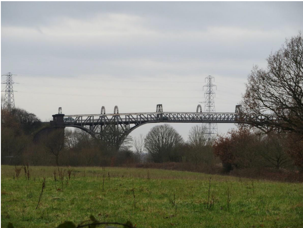
Plate 42 Warburton Bridge, as seen from the SW edge of the Site
