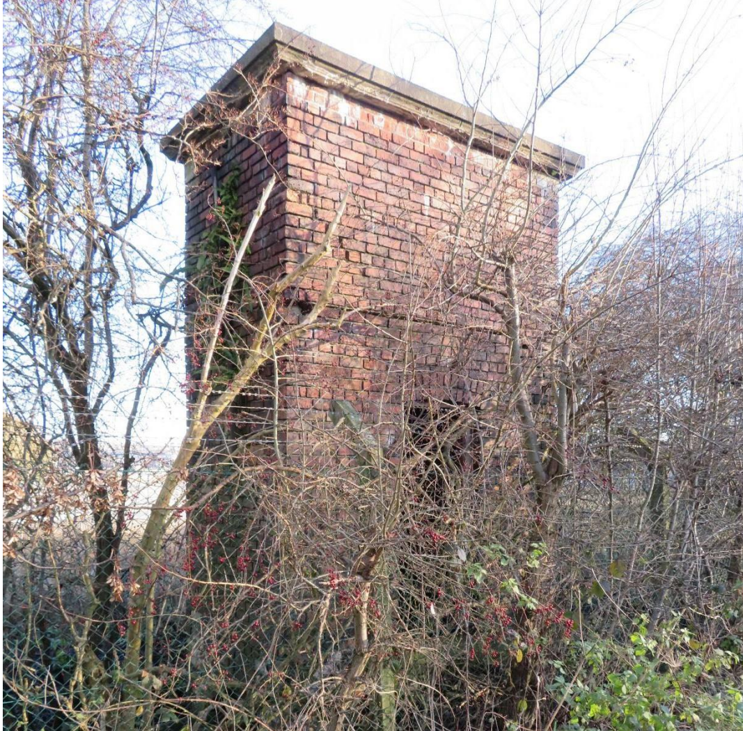
Plate 3 Water Tower on Common Lane to supply the locomotives at Carrington Moss
