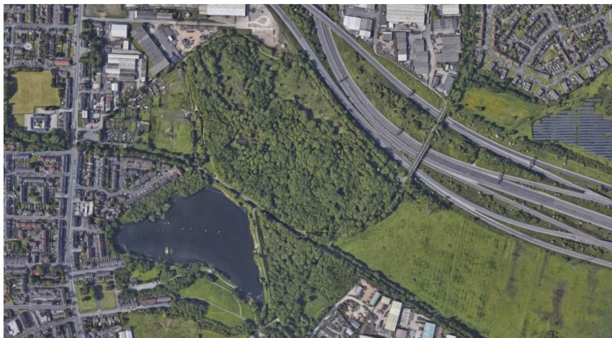
Figure 4 - Aerial view, Blackleach Country Park, Walkden.
