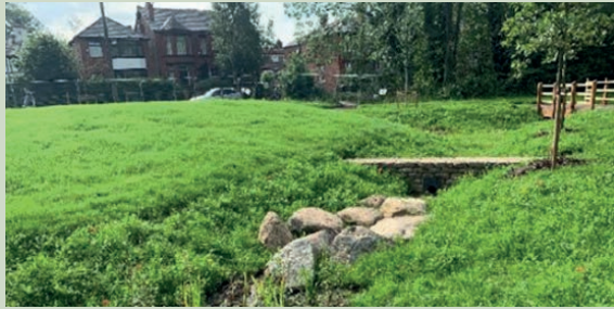
Figure 14 Main swale and check dam flow control feature, showing wetland planting and boulders placed to remove energy from circulating flows.
